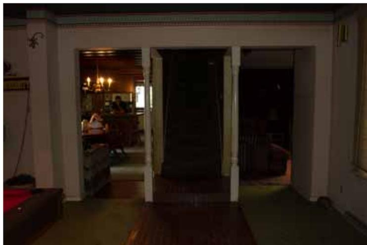
"Before" and "after" shots of the stairway, facing east. Incredibly, those two skinny pillars held up that broad beam! The contractor engineered it so that the beam could be eliminated and the structure made much more solid. While he was at it, he altered the first step to reduce the possibility of tripping.
