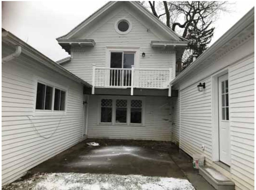
The patio, facing south. There is some damage to the paint on the right of the banquet hall windows, thanks to decades of no gutters. We have full gutters now. Despite being a century old, the wood is in good shape: it's yellow spruce. They built things to last, back in the day.
